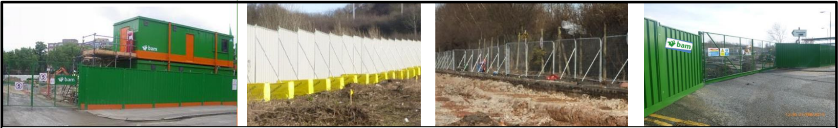
2.4m high solid panel perimeter hoardings supported off kentledge blocks. Heras fencing used for short duration interface works and around access gates for improved visibility.
